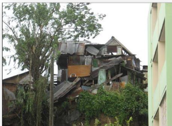
Figure 2: Damage caused by Hurricane Dean, 2007
