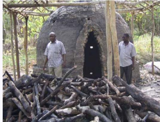
*A Half Orange Brick Kiln constructed in one of the villages under the Dar Charcoal Project*
